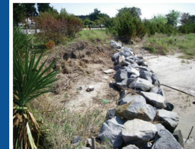
5b. Erosion of bank behind granite rock at upland edge of marsh-sill site on west side of Pivers Island
