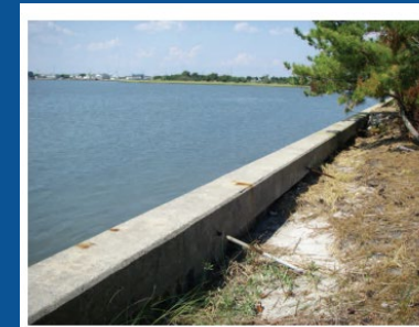
5a. Erosion behind seawall on west side of Pivers Island
